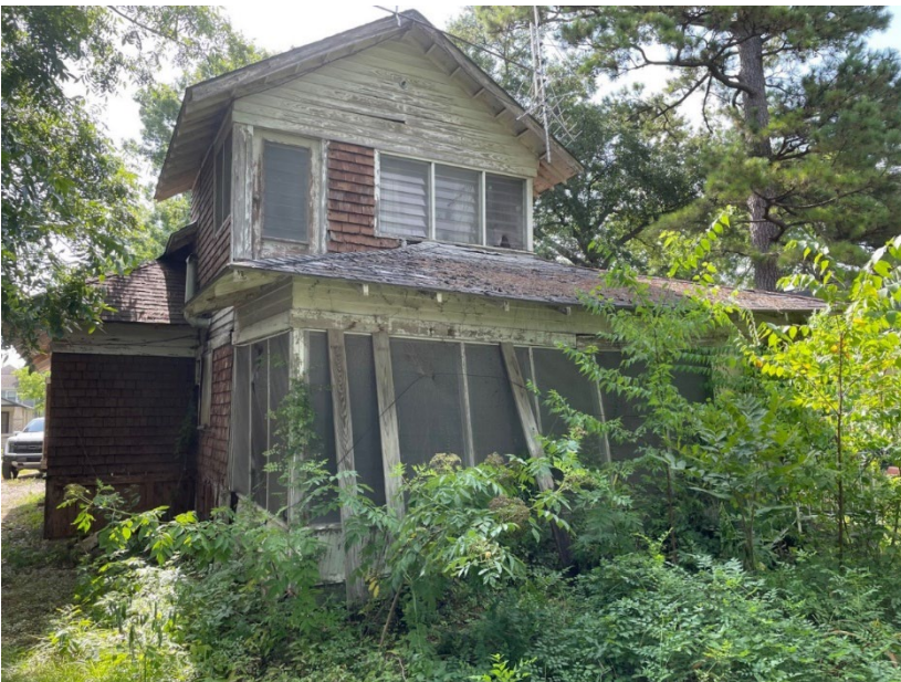
Figure 3- The 2 images above are showing parts of home to be removed.
